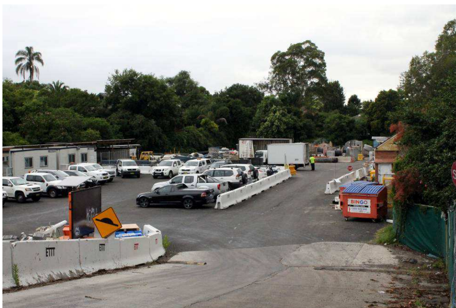
Figure 16 – Works depot for the Epping to Thornleigh Third Track project, located on the site of the former Bowling Club
