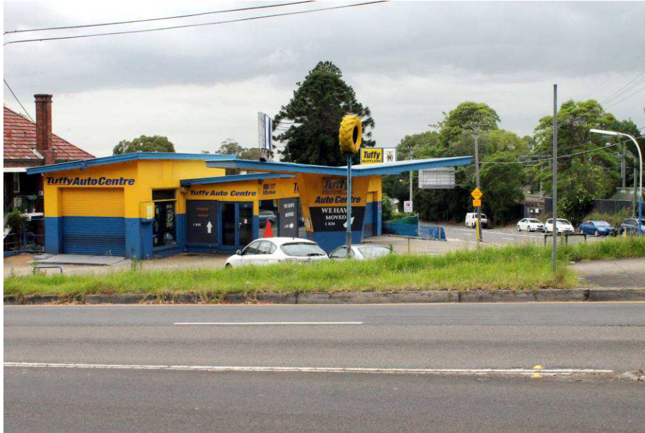
Figure 15 – Former Tuffy Auto Centre workshop
