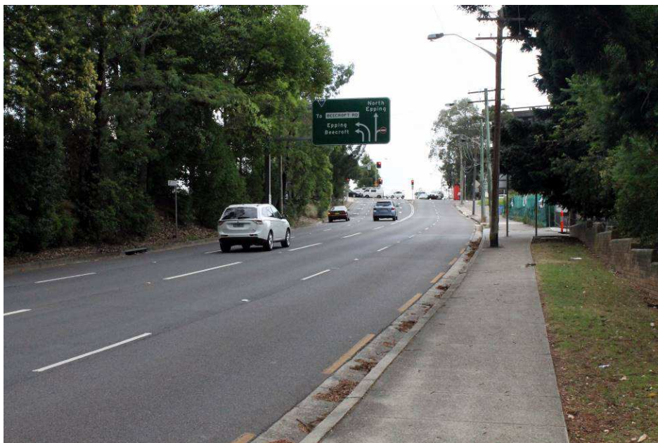
Figure 8 – Blaxland Road, looking north towards Epping Road
