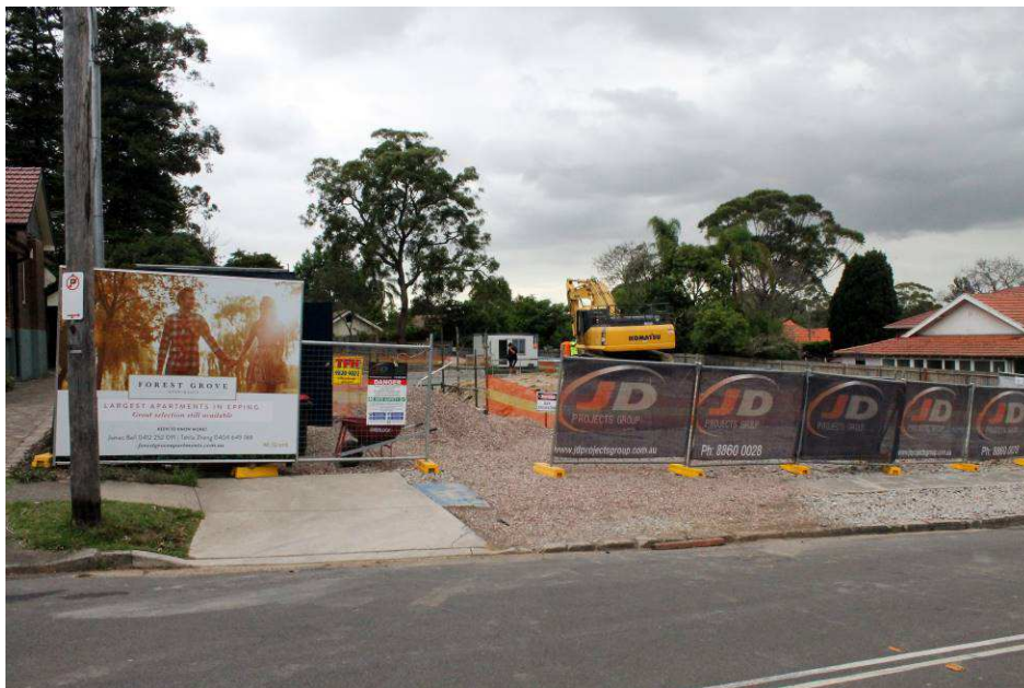
Figure 12 – Residential flat building construction site to the east of Forest Grove
